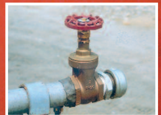
Pipe valve repair carried out using the PlasSteel Twist Stick.
