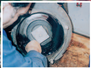
Butterfly valve seam being reinstated using the '80' Durometer Fluid Elastomer.
