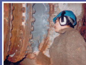
Tank seams repaired using the Extended Life Super Metal Rebuilding System.
