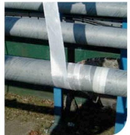
UPS Pipe Repair Bandage TRK 19601/3/4/5
