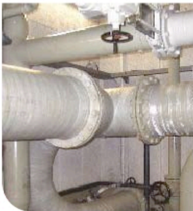
UPS A & B Cement TRK 19002/3
